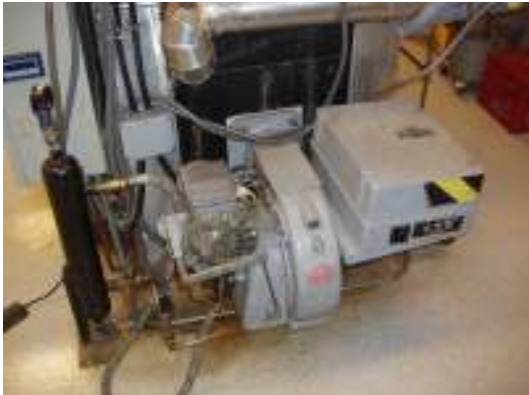
Figure 8: Boiler Burner Assembly
