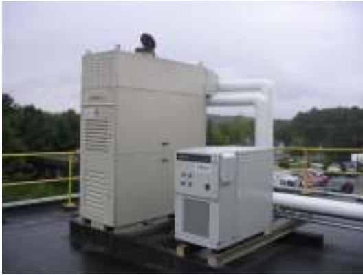
Figure 2: (Capstone 60 kW, CHP unit installed at Quirk auto dealership in Bangor, Maine)
