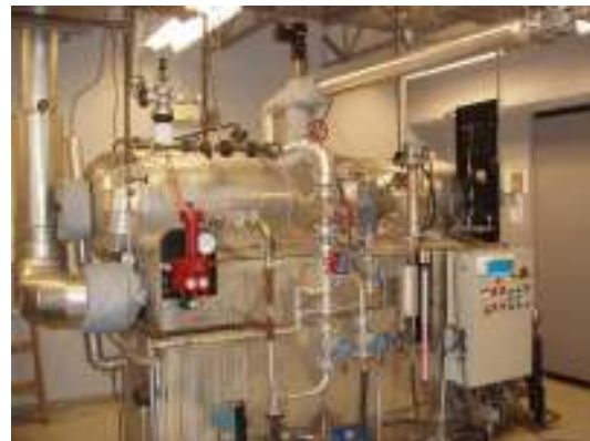
Figure 6: MMA Steam Plant Lab Boiler
