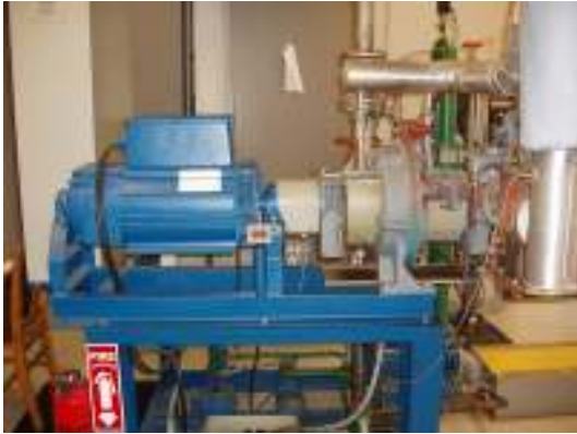
Figure 7: Curtis turbine and Generator
